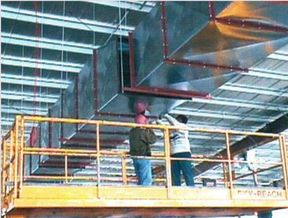
West Point Home Spinning Unit Installation of air conditioning system
