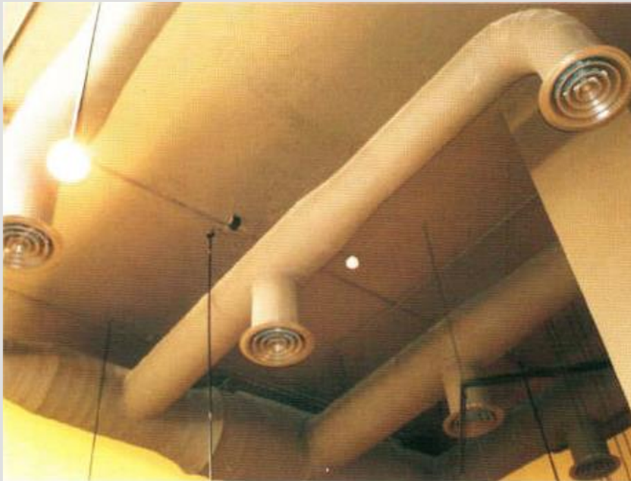
Juffair Skyview Installation of air conditioning system
