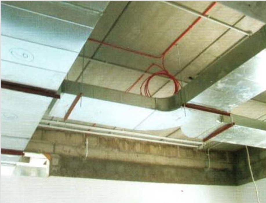
Isa Hadi Engineering (Residential Project) Installation of air conditioning system
