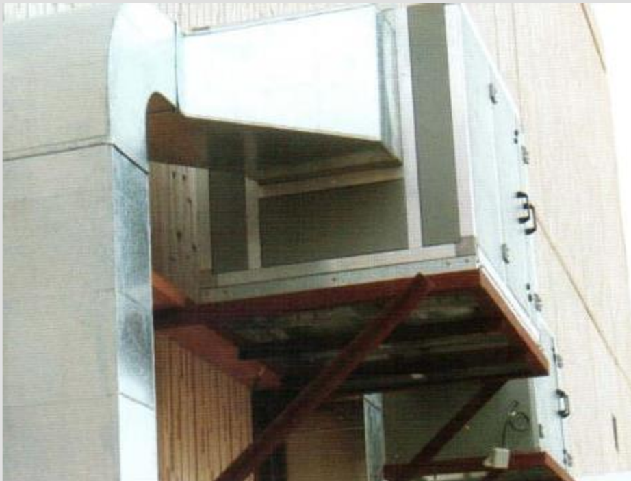
West Point Home Weaving Unit Installation of air conditioning system
